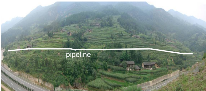
Figure 8. The Erlangmiao Landslide
