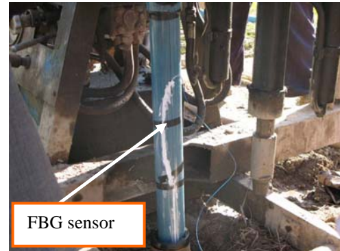
Figure 5. The Pipe Strain Gage Being Inserted to a Bore Hole
